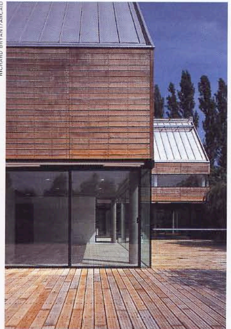
Above left: a perspective drawing of the composite glulam and concrete structure of the Raoul Fonquerne Aquatic Centre in Sète, France. Above: the green oak cladding at David Chipperfield Architects' River and Rowing Museum, Henley-on-Thames.
