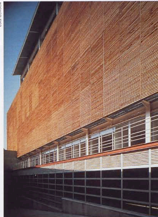
Top: a tubular steel rib structure carries the soaring elliptical vault that roofs Mexico City's National School of Theatre. Above: a slatted screen of California Redwood shades the school's top four storeys.
