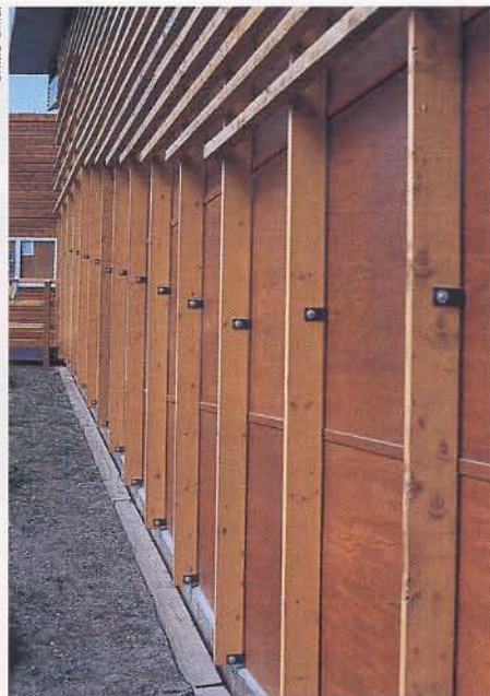
Above left: the Tr'ondek Hwech'in Cultural Centre in Dawson City, Yukon. Above: a detail of the wood lattice screens that refer to traditional fish drying racks. Far left: the random, rough sawn plank cladding on the circular exhibition space recalls Tr'ondek Hwech'in brush huts used for winter shelter. Left: connection details for the rough sawn cladding.
